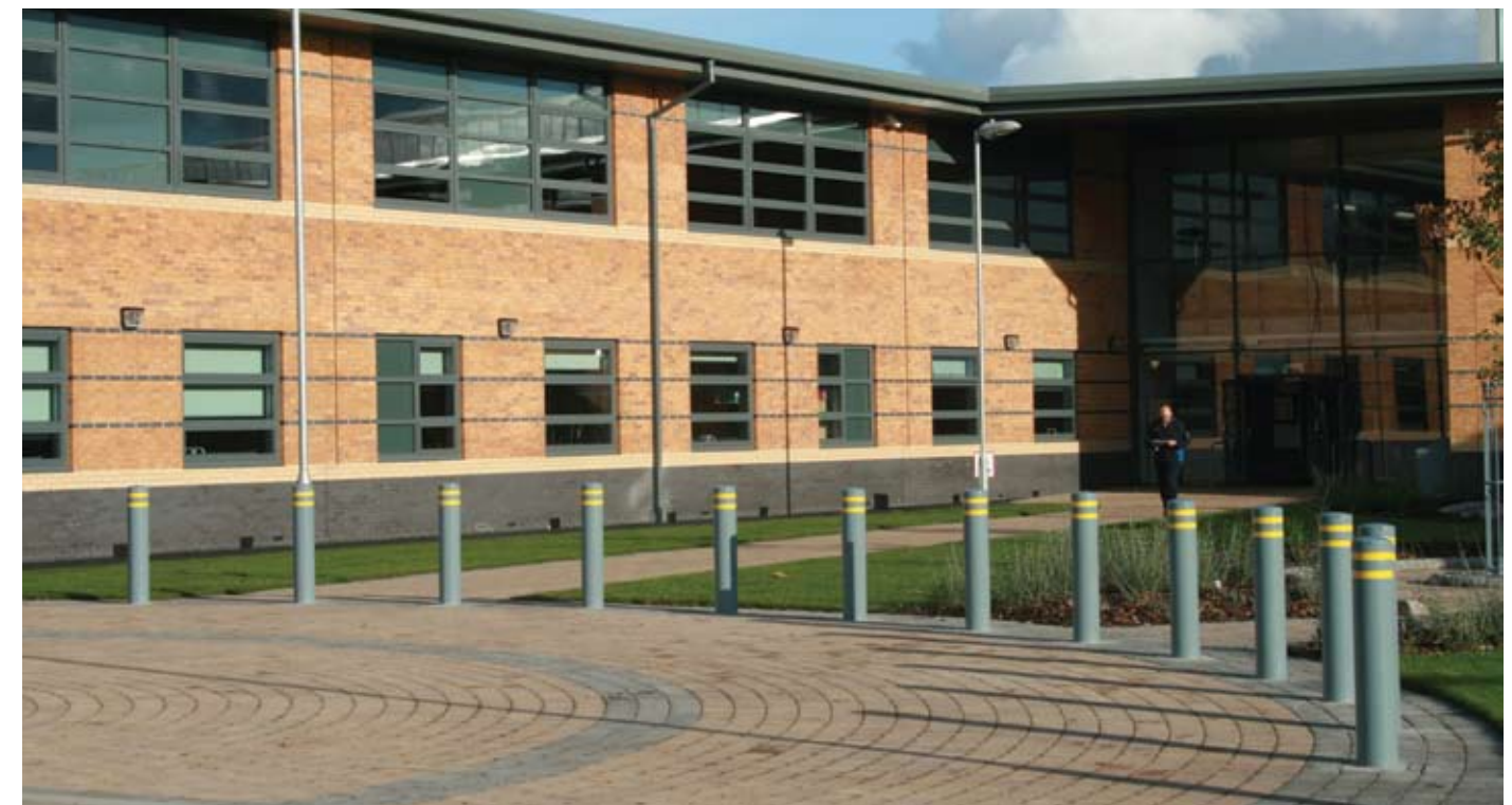
RB 111 Steel Bollards with yellow banding on Tegula block paving in Traditional and Pennant Grey, Harrop Fold High School, Salford
