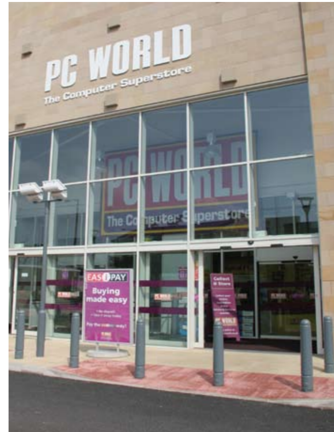
Ferrocast Anti Ram Bollards, PC World, Lancaster
